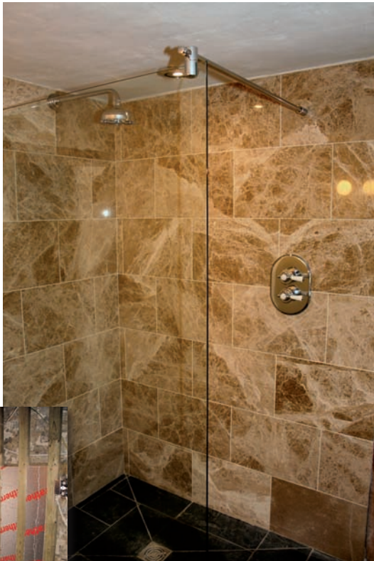
The shower area studwork fitted away from the stone wall with modern insulation between the studs
