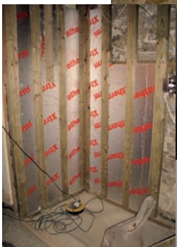
The shower area studwork fitted away from the stone wall with modern insulation between the studs
