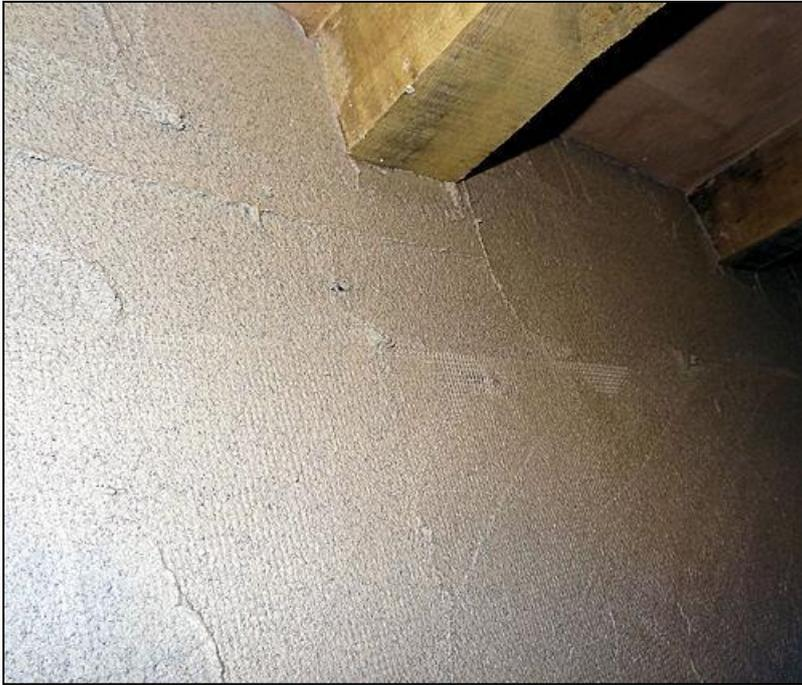
Place a 4mm, 160gm fibre glass mesh across the whole of the wall immediately after notching the AdhereVit and work it in. Add more AdhereVit if necessary. Once the mesh is totally concealed, the AdhereVit should be left for about 24hrs depending on how well the plaster hardens.
