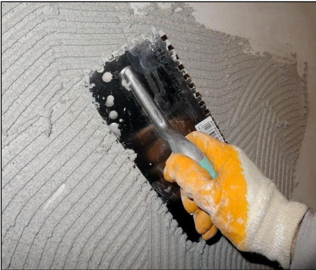
Once any undulations have been levelled, use Secil AdhereVit to fix the board to the wall. The AdhereVit should be notched as this helps to provide the all important all over contact with board and wall without voids or bumps.
