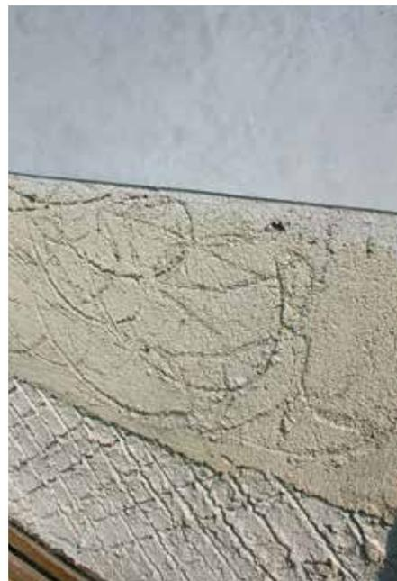
External renders on to solid masonry normally consist of a harl/scat coat, a haired scratch coat and an unhaired float coat (with the addition of an extra dubbing-out scratch coat for very uneven substrates).
